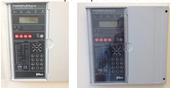
The fire alarm can be activated by smoke & heat detectors and break glass points. The alarm is a siren
