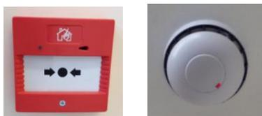
Any faults on the system will cause a buzzer to sound and a fault light to show on the fire panel. The panel will isolate this particular fault. The fire alarm panel will continue to work even if a fault is indicated. The fault should be investigated and repaired with urgency.
